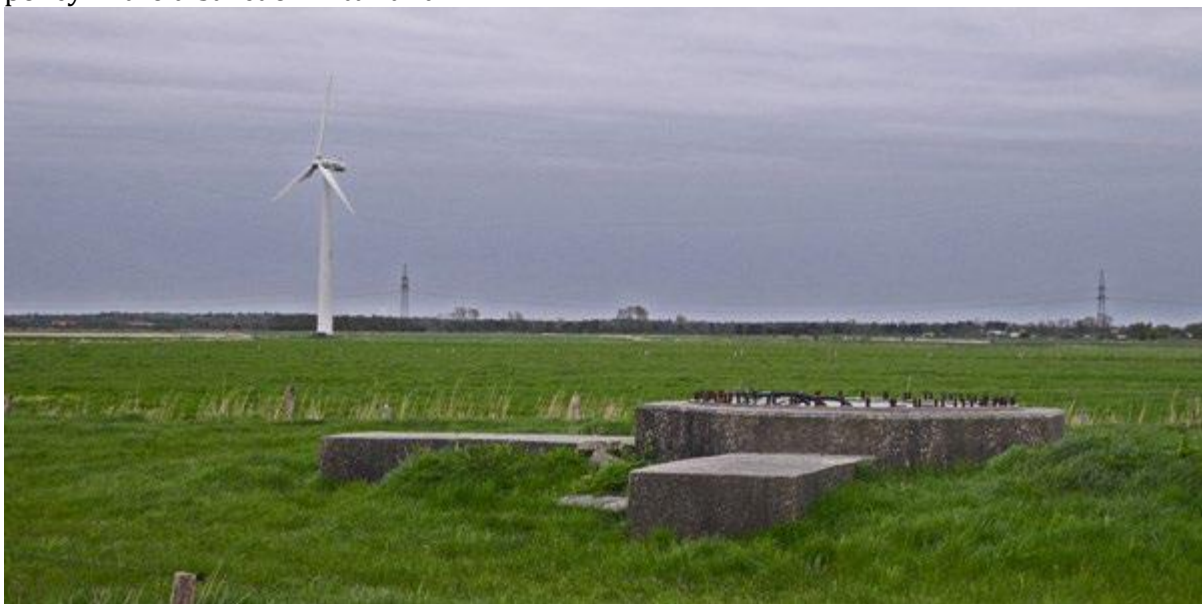
Foundation of the "Zeiger mill" in Oldendorf/Bensersiel, district of Wittmund, which
